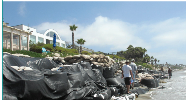
B. Broad Beach, Malibu (2008), with temporary sand bags, which didn't last a single winter and were replaced by a rock revetment (Figure source: Deepika Shrestha Ross).
