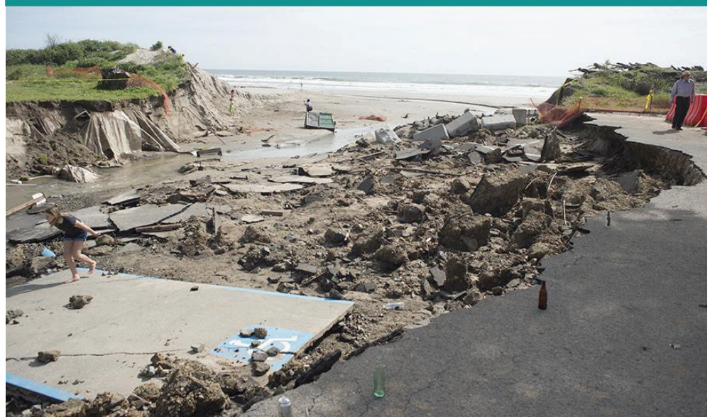
Stinson Beach parking lot closed in 2018 after a storm caused part of it to fall into the ocean (Figure source: David Briggs, The Point Reyes Light).
