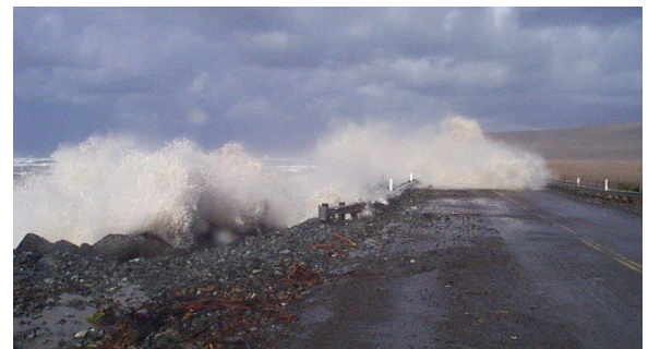
California Highway 1 before realignment with high swells, San Piedras. (Figure source: Caltrans).
