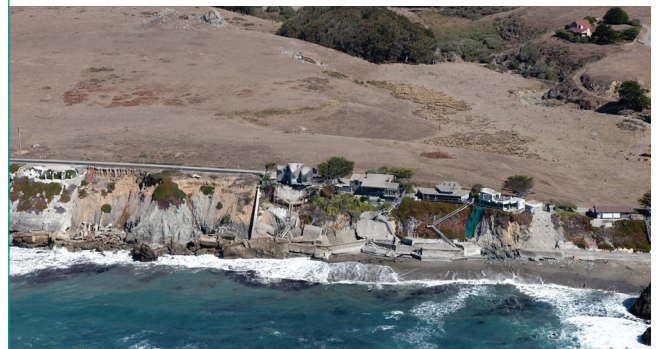
B. Gleason Beach, Sonoma County, where most of the homes have now been destroyed or removed (2009; Figure source: Kenneth and Gabrielle Adelman, California Coastal Records Project, www.Californiacoastline.org ).
