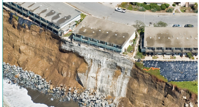
B. The same apartment buildings in Pacifica shown in Figure 5A in 2011 with failure of protection efforts prior to demolition (Figure source: Joel Avila, Hawkeye Photography).
